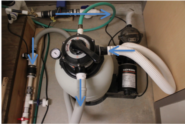
Figure 3.6 Hayward Pressure Sand Filter
