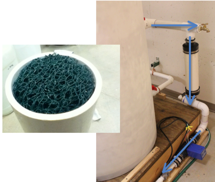
Figure 3.5 Coarse Matala Filter
