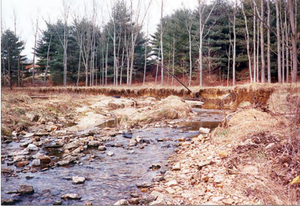
FIGURE 3. Pre-restoration photograph of Minebank Run (2003). View looking upstream from the confluence with the Harts Run tributary at the upstream end of the study reach. Image courtesy of U.S. Geological Survey Scientific Investigations Report 2012-5012.
