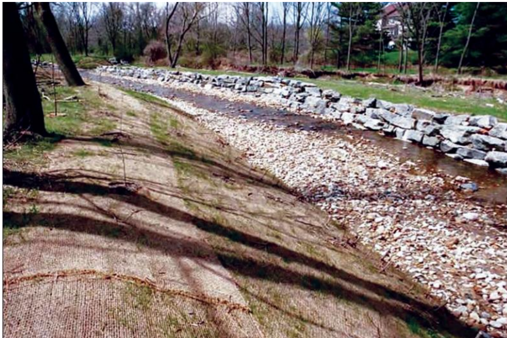
FIGURE 4. Restored section of Minebank Run (2005). View looking upstream from the confluence with the Harts Run tributary at the upstream end of the study reach with the original channel visible in the background. Image courtesy of U.S. Geological Survey Scientific Investigations Report 2012-5012.
