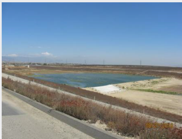
FIGURE 6-5-1 Regional stormwater recharge in the Chino Basin. SOURCE: Rich Atwater.
