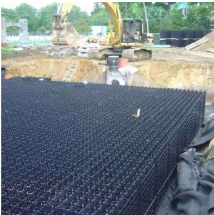
FIGURE 6-7 Subsurface stormwater storage under construction for the Darien Library (a LEED Gold facility) in Darien, Connecticut. The tank holds 83,500 gallons. SOURCE: http://www.invisiblestructures.com/project_profiles/page/2 .
