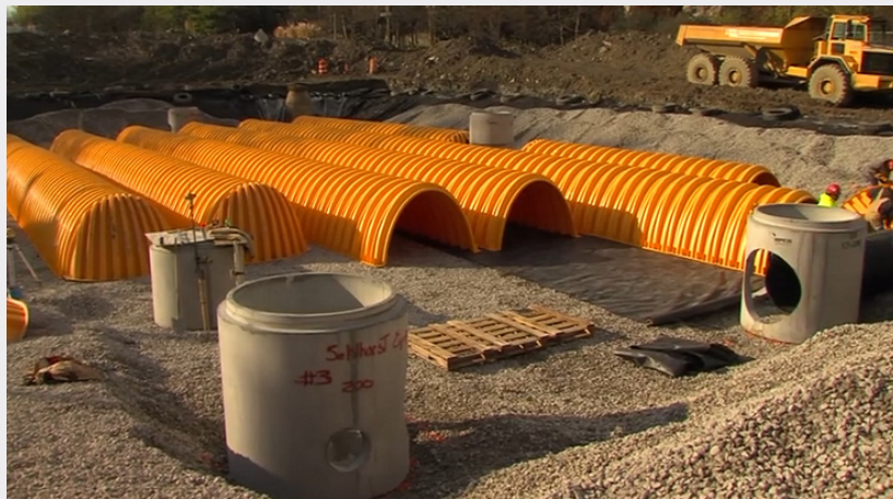
FIGURE 2-3-1 Construction of subsurface stormwater storage at the Cincinnati Zoo (top). SOURCE: http://www.youtube.com/watch?v=6SJLraXsxys .
