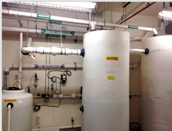
FIGURE 2-2-1 Storage and treatment system for the graywater toilet flushing system at Aspen Residential Hall, Colorado State University. SOURCE: Courtesy of Sybil Sharvelle.
