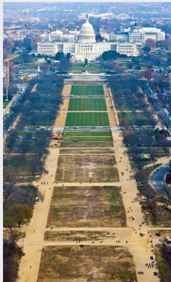
FIGURE 2-5-1 Phase 1 of the National Mall turf restoration project rehabilitated eight lawn panels between 3rd and 7th Street, NW, and installed 500,000 gallons (2 million liters) of stormwater storage capacity. SOURCE: M. Stachowicz, NPS, personal communication, 2014.
