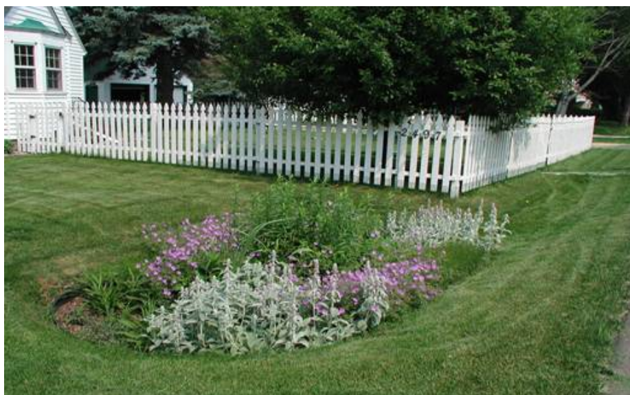
FIGURE 6-12 Household-scale rain garden. SOURCE: https://www.bae.ncsu.edu/topic/raingarden/stormwater.htm .
