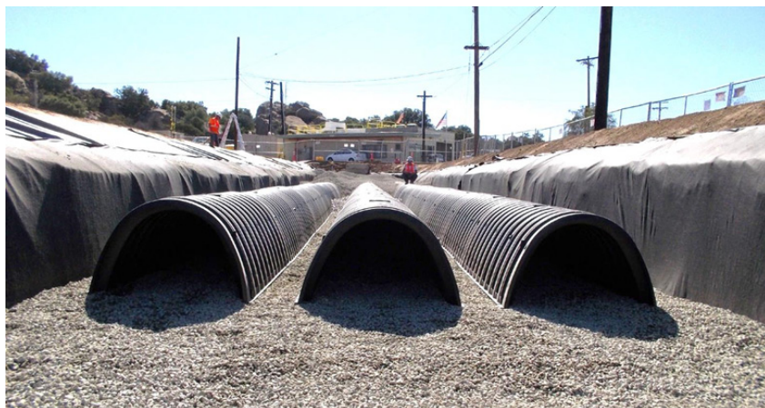
FIGURE 6-14 Biofilter/swale under construction with underground water storage vaults for irrigation use. SOURCE: Photo by Dan Bourdeau, Geosyntec, Inc.
