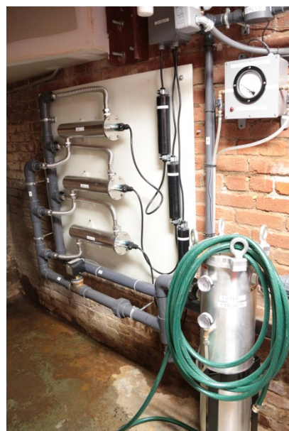
FIGURE 6-9 Small on-demand water treatment system with ultraviolet (UV) disinfection used to treat roof runoff for vehicle washing at a Washington, DC, fire station.
