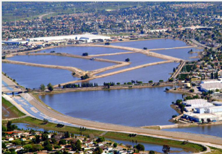
FIGURE 1-4-1 Rio Hondo Spreading Grounds, which receives controlled releases from San Gabriel Canyon, Santa Fe, and Whittier Narrows dams for groundwater recharge. SOURCE: http://www.wrd.org/engineering/groundwater-replenishment-spreading-grounds.php .
