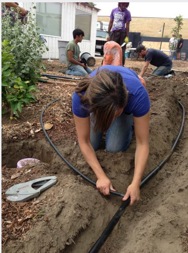
FIGURE 2-3-1 The City of Long Beach piloted a laundry-to-landscape graywater program at 33 homes to assess costs, homeowner satisfaction, and water savings. Laundry water is conveyed directly from a clothes washer via buried pipes to drip irrigation systems. SOURCE: Photo courtesy of Jason Gallup, Office of Sustainability, City of Long Beach.
