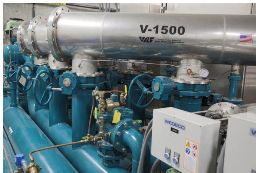
FIGURE 6-11 Large stormwater treatment system underground of the Washington, DC, mall, designed to treat stormwater from tanks holding 1 million gallons (3.8 million liters) for spray irrigation.
