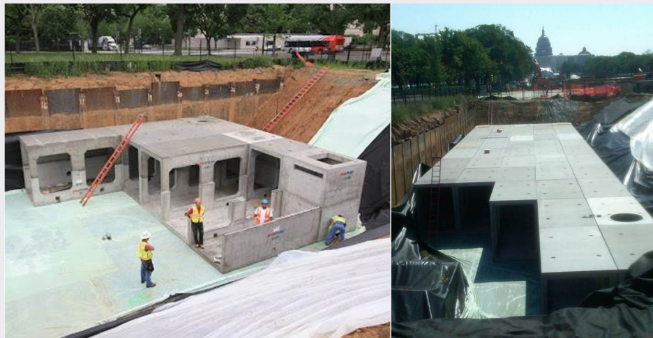
FIGURE 2-5-2 Installation of a 250,000-gallon (950,000-liter) cistern beneath the National Mall in Washington, DC. The captured stormwater is used to irrigate the turf along the National Mall. SOURCE: M. Stachowicz, NPS, personal communication, 2014.
