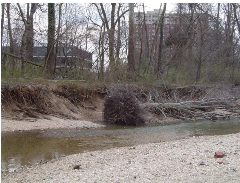
FIGURE 1-7 Urbanization has increased stormwater runoff in Paint Branch, in College Park, Maryland. The resulting hydromodification causes more erosion, deepening of urban streams, and unstable channels compared to the pre-development state. SOURCE: http://www.anacostiaaws.org/news/blog/tags/12 .
