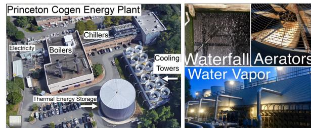
Figure 2. Left side: Overview of Princeton's energy plant. Right side: A dozen cooling towers use aerators and a waterfall perimeter to reduce the temperature of hot water from ~95°F to surrounding air temperature, emitting water vapor in the process.
