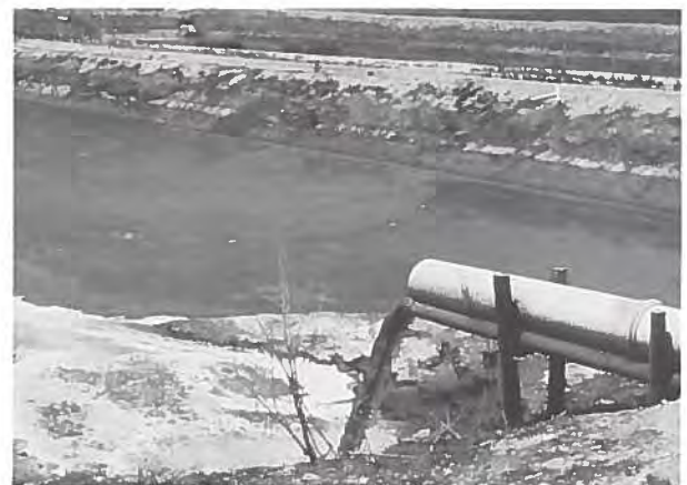
Liquid waste holding structure
