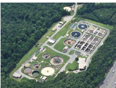
North Cary Water Reclamation Facility achieves nutrient removal with a Kreuger Bio-Denitro Process (oxidation ditch w/BNR) and receives nutrient credit for effluent water reuse. (Photo credit: www.lnba.net)
