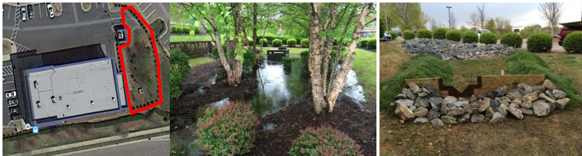
Figure: Aerial photo of Discount Tire (left); main cell with outlet structure (center); inlet from parking lot (right)
